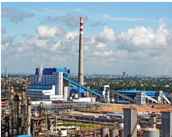
SINOPEC Maoming 2 x 100 MWe CFB
