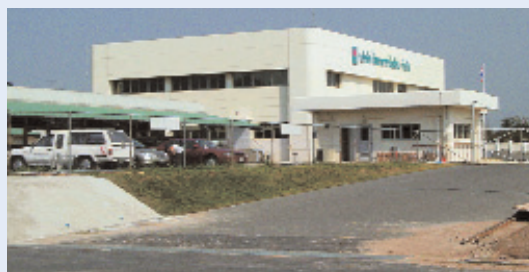
TPX administration building.
