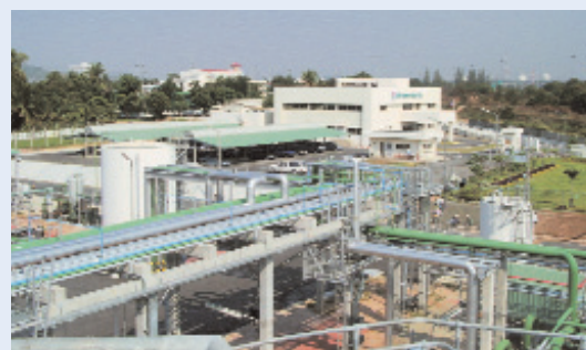
Utilities units located to south of the process units, with TPX administration building in the background.
